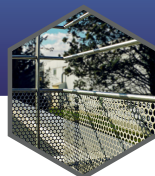
GARDE CORPS PUBLIC
